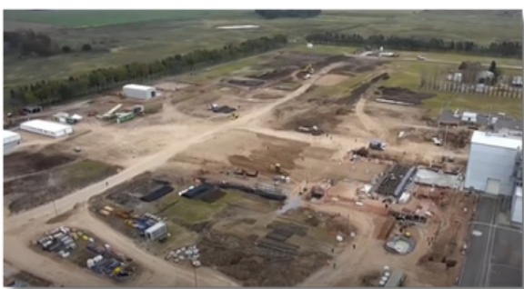
Remote Inspection Construction Site
